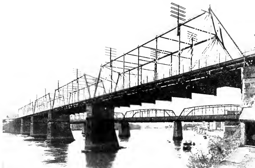
THE BOSTON & MAINE RAILROAD BRIDGE—COUNTY BRIDGE IN THE BACKGROUND
